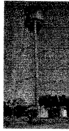
City Water Tower
